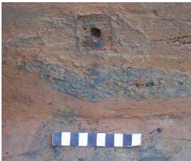
Figure 8. Imprint of corroded iron fastening. (Victoria Tomalin)
